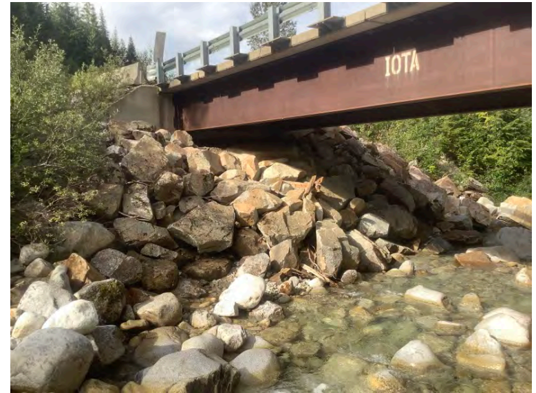
Left Bank Abutment when facing downstream
