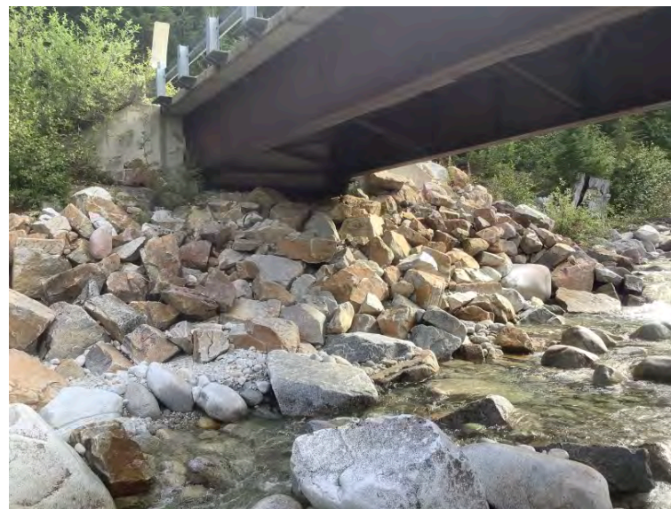
Right Bank Abutment when facing downstream
